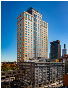
Our first adaptive reuse project in more than two decades, 90 Sands is a conversion of a former residential hotel into 491 units of permanent supportive and affordable housing. 305 apartments are set aside for individuals exiting homelessness, and the balance of 186 units are home to low-to-moderate income households. Situated in one of Brooklyn's most expensive neighborhoods, 90 Sands also provides extraordinary views of lower Manhattan, Brooklyn, and all the way to Queens.
